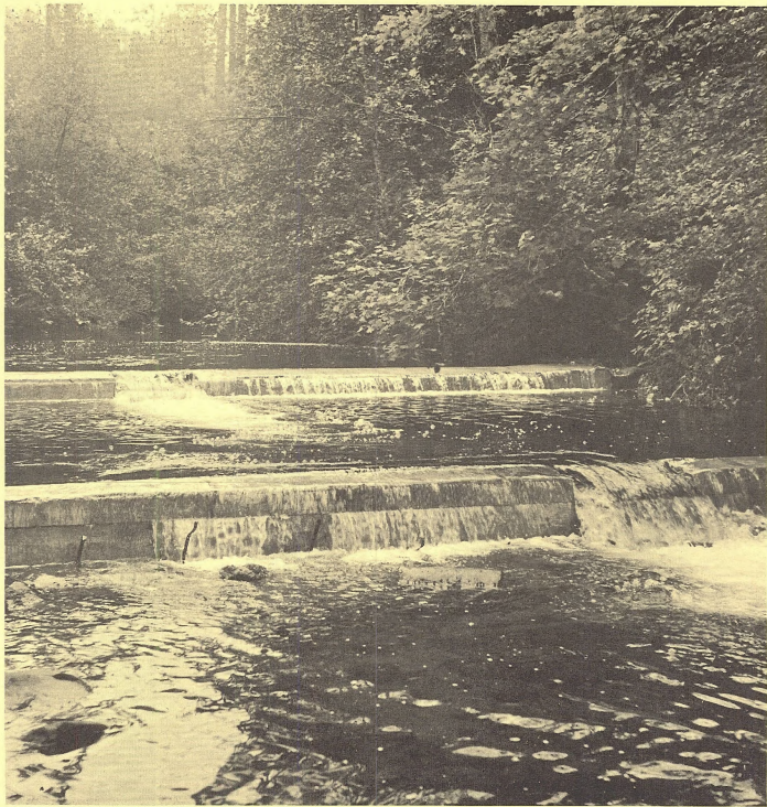
Illustration 4 - View of West Branch of Smith River after dams were completed. Form iron was removed after photograph was taken.
